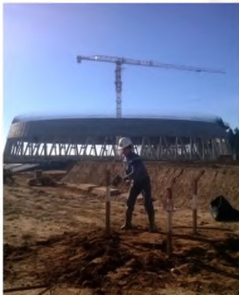
Working on a Belarusian Power Plant site
