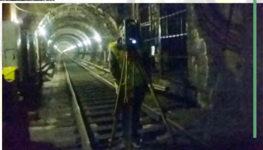
Monitoring of deformations of the metro tunnel in Minsk, Belarus
