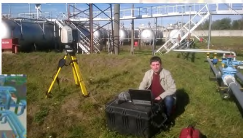
3D scanning of a gas filling station
